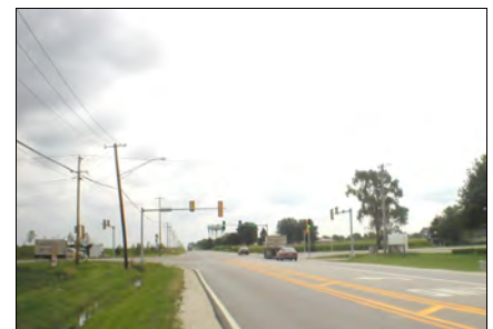
Laraway Road at IL 53
