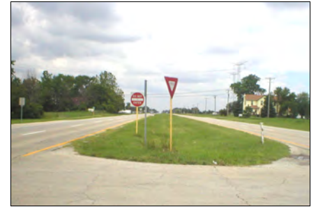
Illinois Route 53 at Millsdale Road
