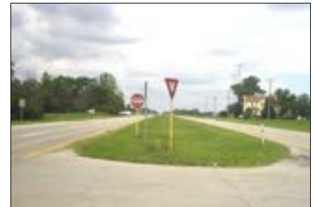
Illinois Route 53 at Millsdale Road
