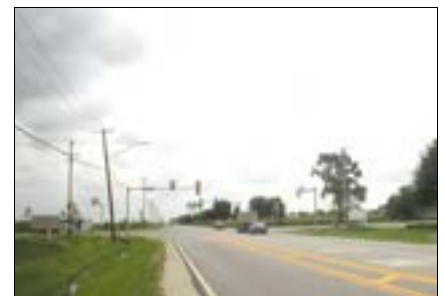
Laraway Road at IL 53
