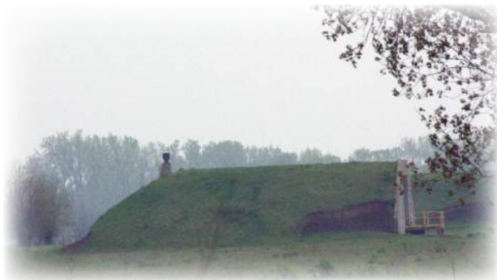
One of 392 igloos used to store munitions at the JOAAP.
