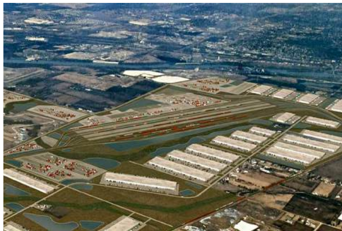
CenterPoint Intermodal Center - Joliet
