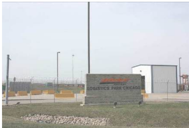
Entrance to BNSF Intermodal Yard - Elwood
